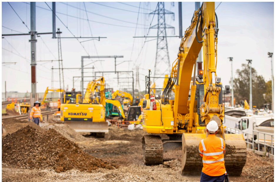
Excavators preparing ground for track turnouts leading into the approach structure at the western portal for the Sunbury Line Upgrade.
