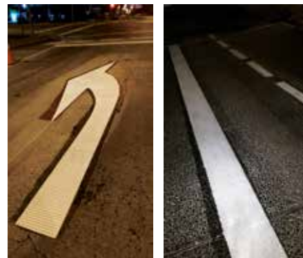
NEWELL HWY FRESHLY INSTALLED UA3, TF3 AND PCW LINES 13/05/2015.
