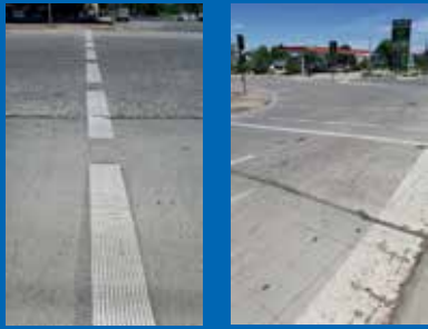
NEWELL HWY AT 18 MONTH INSPECTION 15/11/2016 TF3 AND PCW LINES. NOTE PAVEMENT WEAR.
